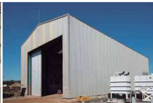
cabine de pintura painting cabin
