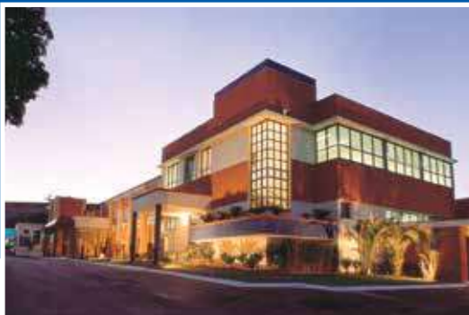
sede administrativa headquarters
