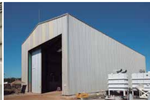
cabine de pintura painting cabin
