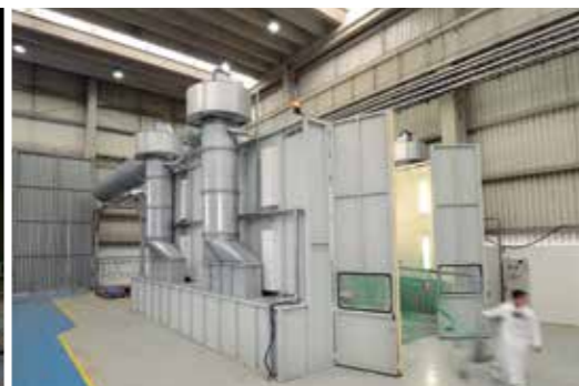
cabine de pintura líquida liquid painting cabin ("cross draft")
